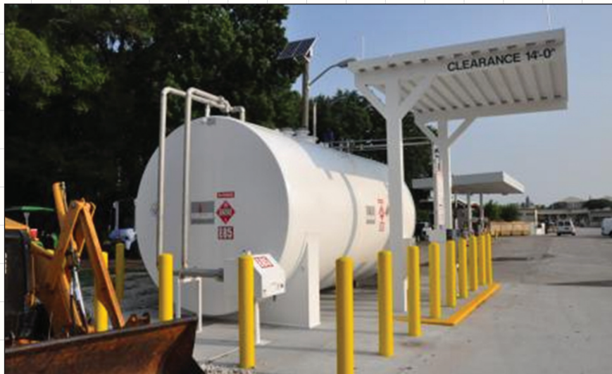
University of Central Florida's E85 fueling station. Source: University of Central Florida.
