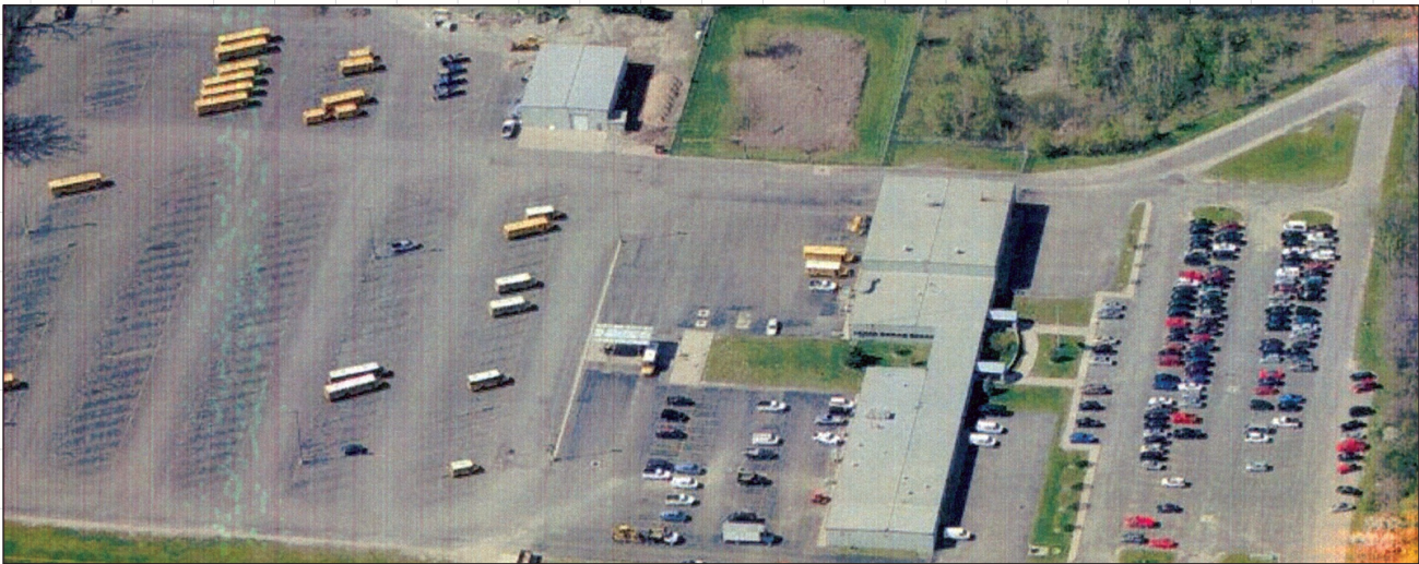
Aerial view of fleet facilities. Photo Courtesy of Jill Segal.
